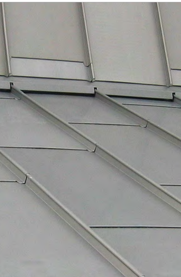
PMR & PMG DOUBLE SEAMED ZINC ROOF TO BUILDING ONE FINISH: RHEINZINK, PATINA LINE, BLUE GREY ZINC HTTPS://WWW.RHEINZINK.COM/EN/PRODUCTS/ROOF-SYSTEMS/ROOF-COVERING-SYSTEMS/DOUBLE-STANDING-SEAM/
