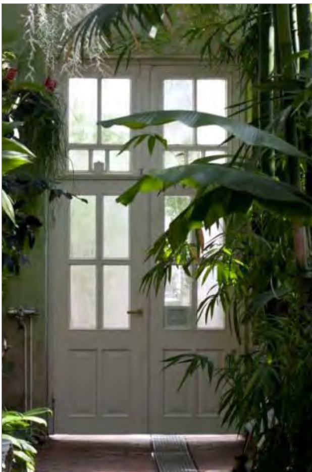
PTD TIMBER DOOR TO BUILDING TWO FINISH: DULUX HIGH TEA GREEN S25B7
